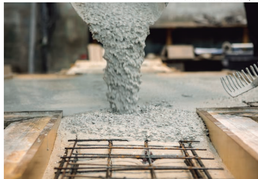
Foto: BASF Construction Chemicals España
