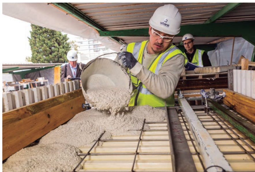
Foto: BASF Construction Chemicals España
