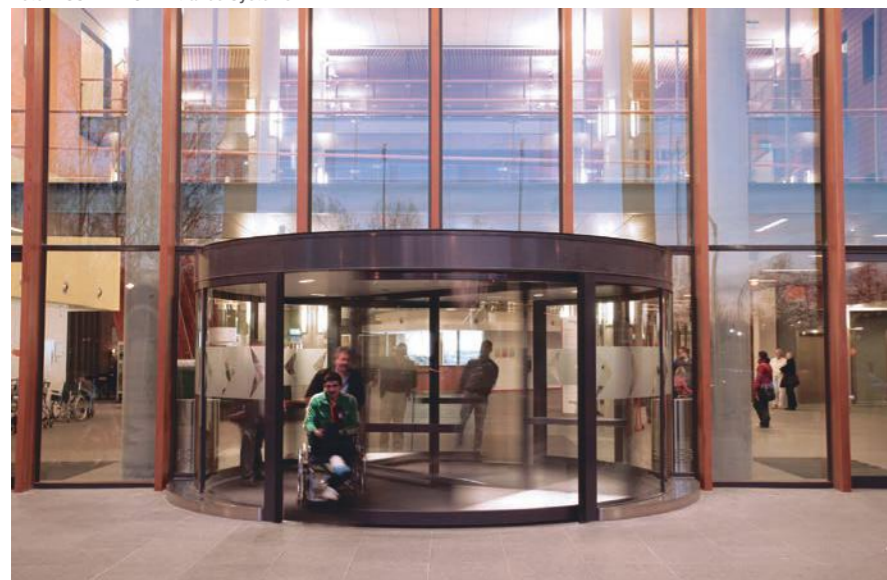
Foto: ASSA ABLOY Entrance Systems
