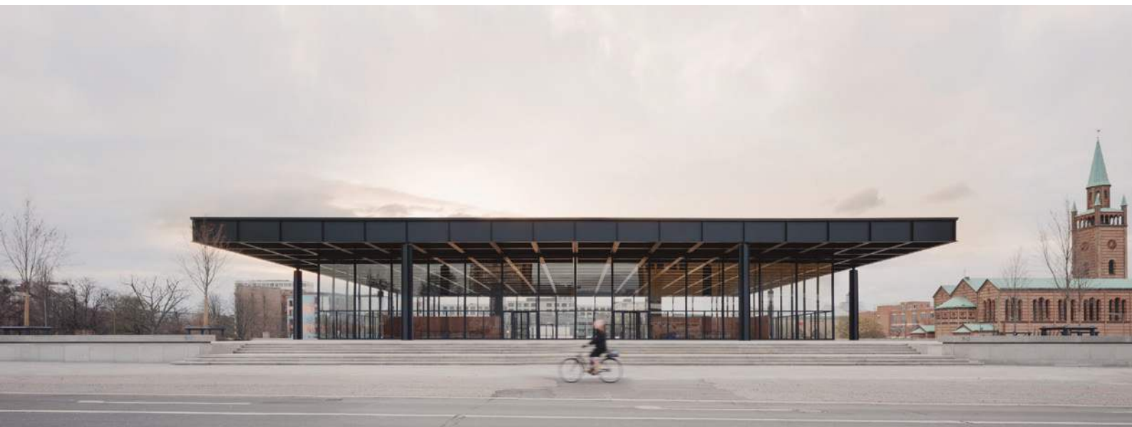
^ Foto: Neue Nationalgalerie refurbishment
